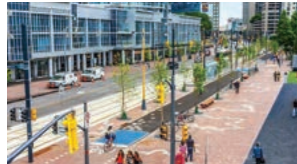
Queens Quay Boulevard, Toronto. Photo credit: City of Toronto.
